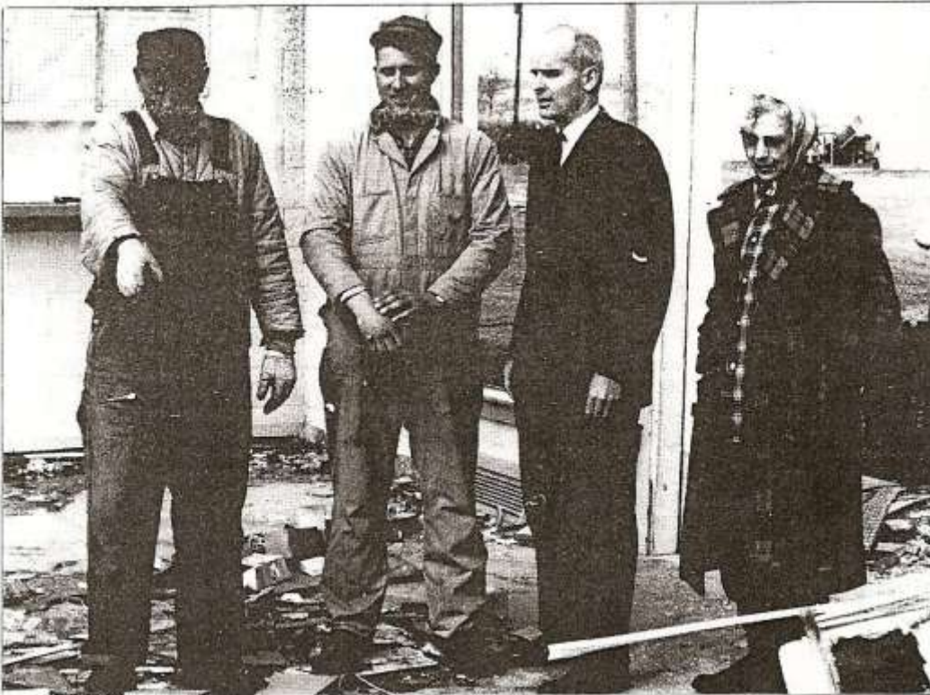
Mrs. J. B. Larsen views the damage that was done by the April 11 tornado to the gift shop and other buildings at the J. B. Larsen Orchard near Evansville. The men in the picture are Senator William Proxmire, right, who was in this area Saturday inspecting the storm damage and Wenzel Renvick and Don Woodstock.
