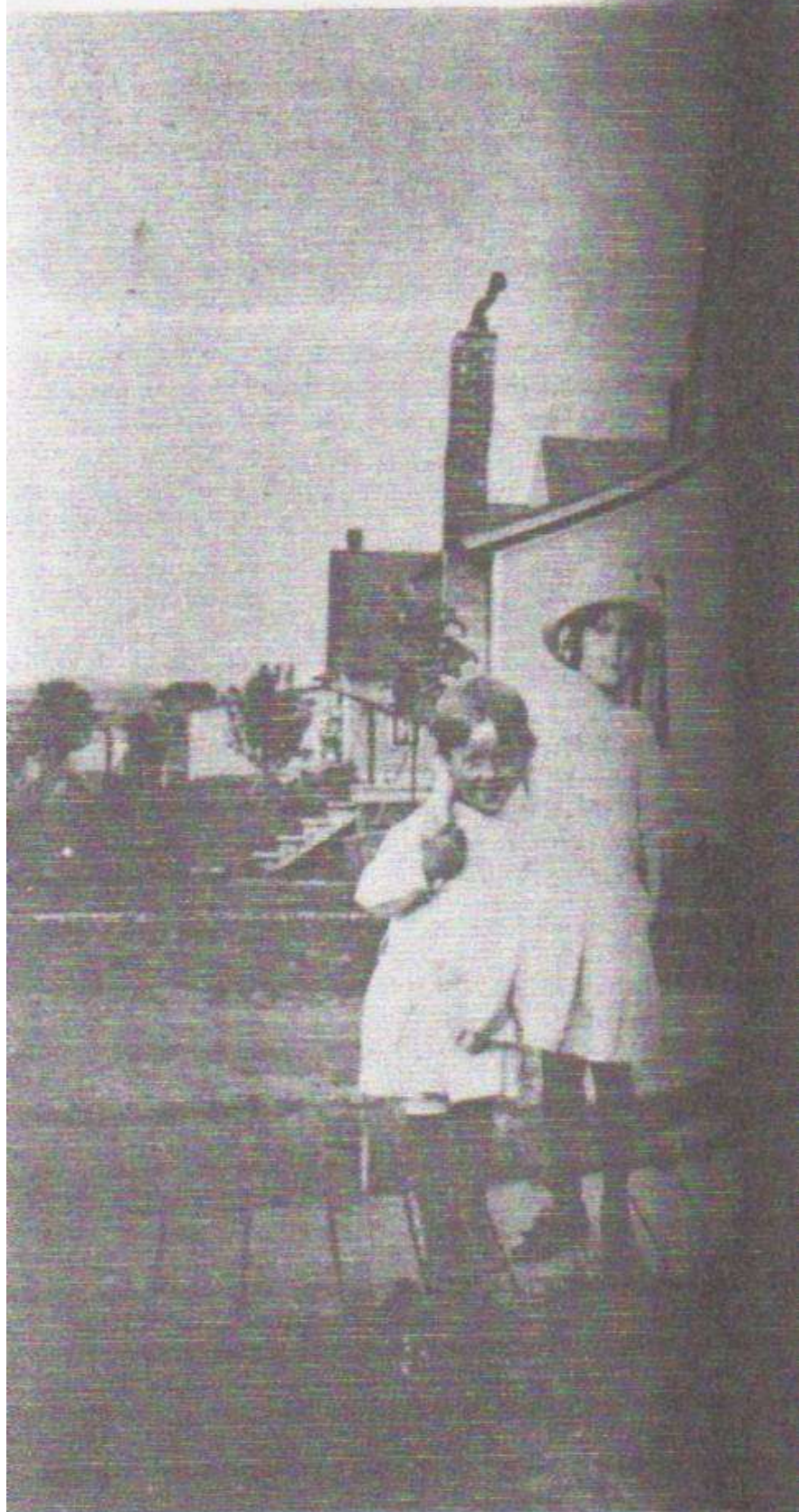
Remember way back when . . . when there were sidewalks with cement sidewalks. Back when the sidewalks were wood. This is a photo taken at the corner of Maple and Washington around 1916. Wayland Cushman and his sister, Mary.
