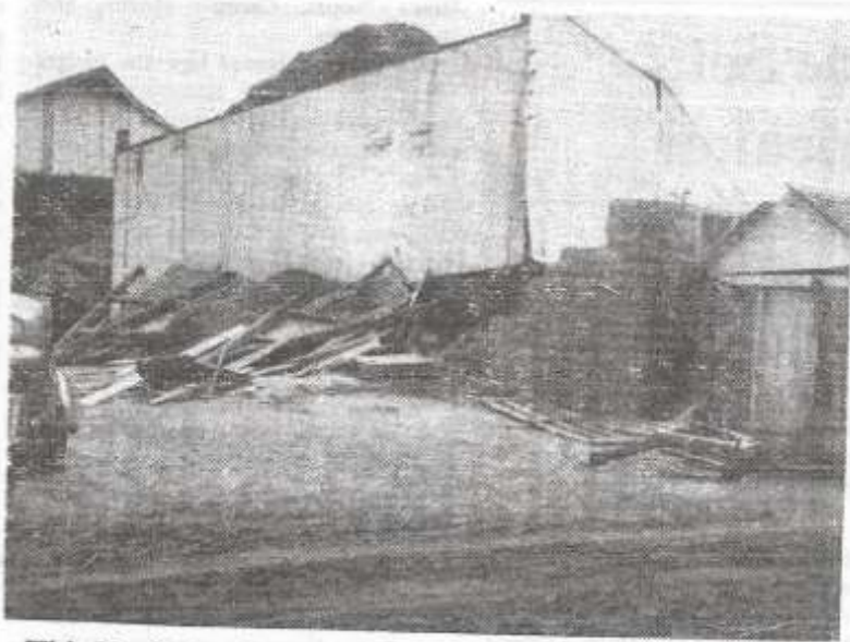
This 30 x 90 foot barn on the Elmer Allen farm was almost completely destroyed by the gale winds that swept through this area causing heavy damage the night of May 20.
